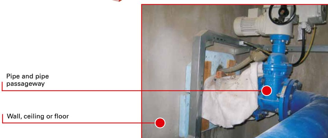
For narrow gaps and cracks, **ERGELIT-superfix 10** is the water-tight, permanent grout that holds the pipe firmly in position where it runs through the wall, in less than 45 minutes.
