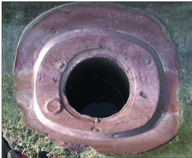
Hächler Umwelttechnik has been partners with ERGELIT in Germany since 1995. ERGELIT supplies the fiber-reinforced mortar to seal the laterals, such as the one shown here.
