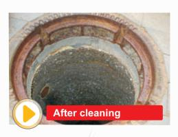
The walls of the shaft are inspected after cleaning. Any possible leaks are sealed off or damaged areas are repaired, using techniques such as pressurised grouting, injection or super-fast **ERGELIT grouts**. All equipment required for this is included as standard in the **M-COATING** system.
