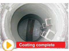
The coating process is based on an integrated system consisting of a mixer, a pump and a centrifugal spray. All three components are fully automated. For loading the grout or controlling the mixer and pump, only one operator is needed.
